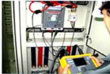
POWER MEASURING & HARMONICS
