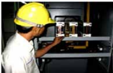
BUSBAR SUPPORT INSPECTION
