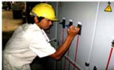
CIRCUIT BREAKER INSPECTION
